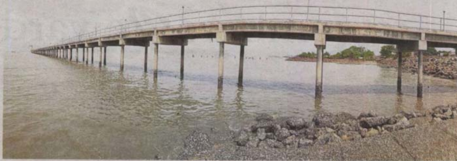
The newly upgraded Lovers' Bridge in Taman Tanjung, Tanjung Sepat.
